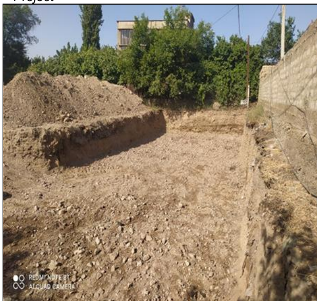
Photo 5: Construction of foundation pits, August 2022
