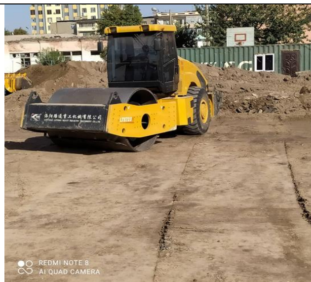
Photo 2: Compacting soil for foundation, August 2022
