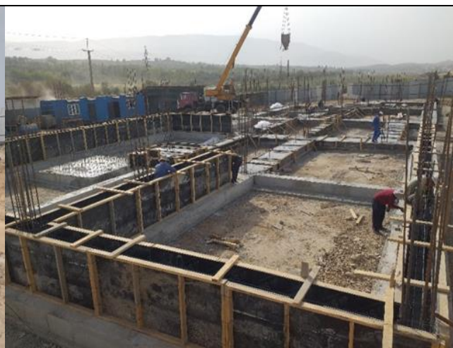
Photo 14: Preparation of formworks for foundation of main building, October 2022
