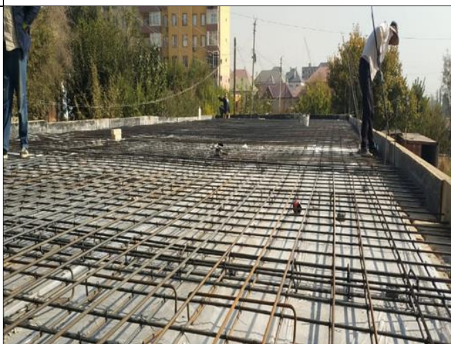
Photo 8: Reinforcement installations for the monolithic slab in the Workshop building, worker not equipped with PPE, September 2022
