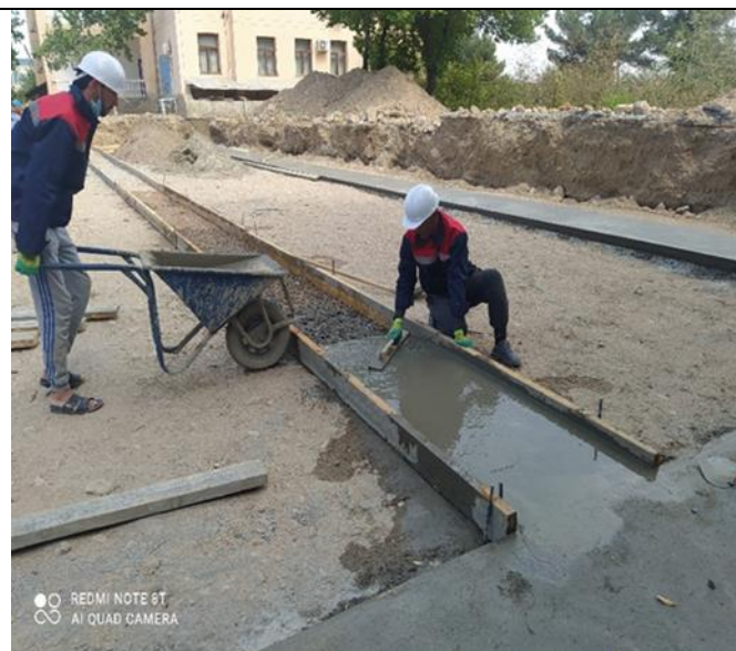
Photo 6: Foundation arrangement, some workers don't wear PPE, September 2022
