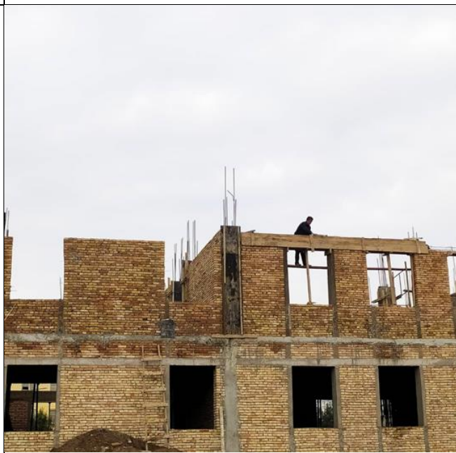
Photo 4: Brickwork on second floor of educational building, November 2022
