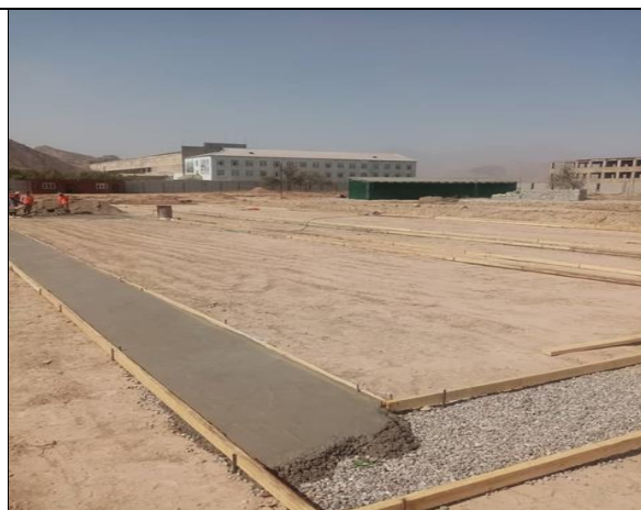
Photo 10: Construction of concrete base for foundation of Dormitory building, September 2022
